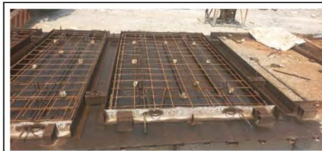
Date Pre Concrete: 7/15/2024
